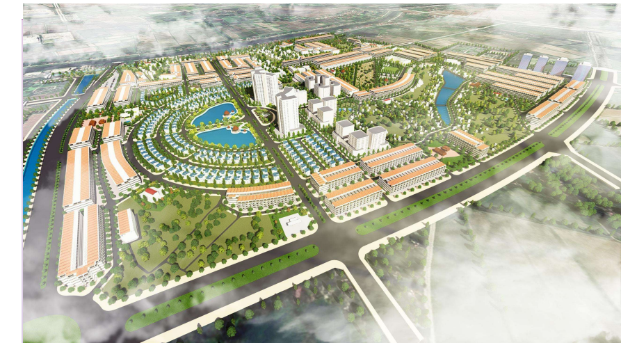
Investment Project for Construction of Tan Ha Residential Area (Phase I)
