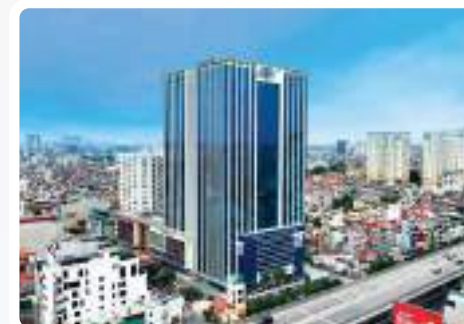
VINACONEX DIAMOND TOWER
